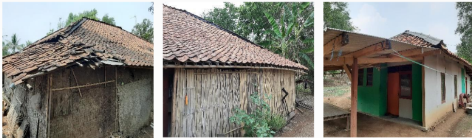
Figure 3. House Condition in The Study Location
