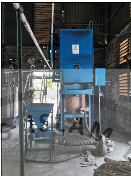
Gambar 4.8 Boiler Vertikal
